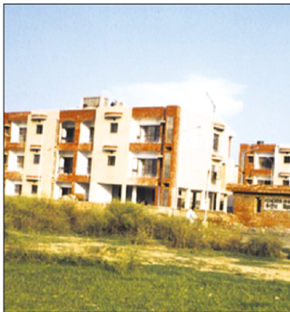
Chandigarh : 305 DUs Completion Year : May, 2000
