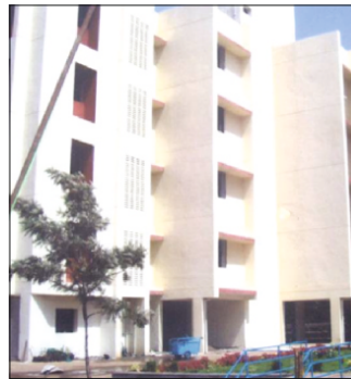
Pune, Ph-II : 148 DUs Completion Year : December, 2008
