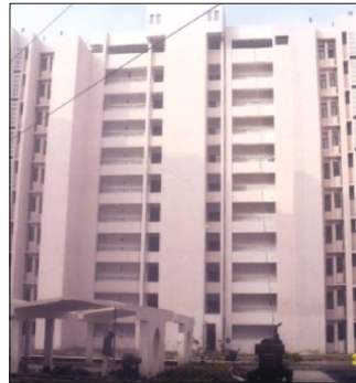
Mohali, Ph-I : 603 DUs Completion Year : April, 2013
