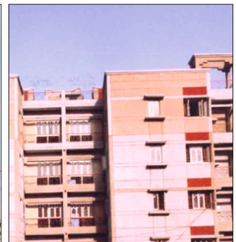
Gurgaon, Ph-I : 1088 DUs Completion Year : July, 1999
